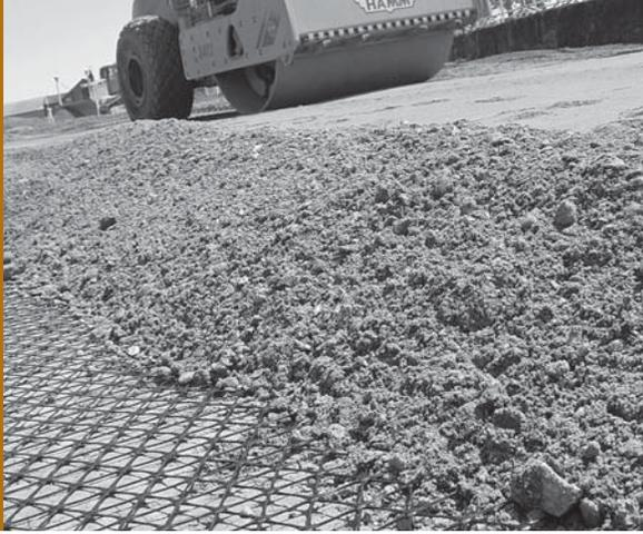
**Image 10** Compacting the aggregate fill.
