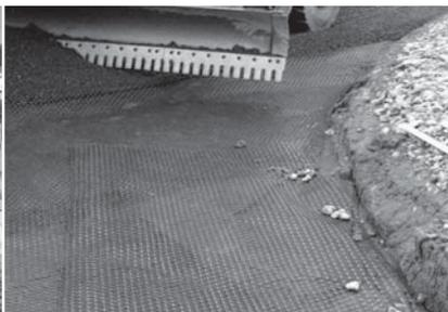
**Image 4** Placing Tensor TriAx Geogrid to accommodate curves.
