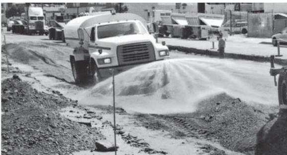
**Image 9** Moistening the fill before compaction.
