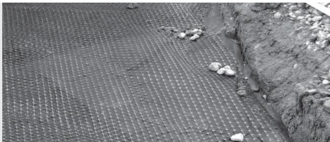
**Image 6** Tensor TriAx Geogrid anchored with small piles of aggregate.
