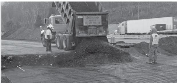
**Image 7** End dumping aggregate fill on top of Tensor TriAx Geogrid over soft subgrade.
