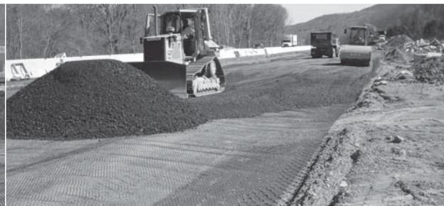
**Image 8** Spreading aggregate fill over Tensor TriAx Geogrid.
