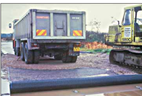
Figure 1: Simple practical demonstration of the benefits of Tensar biaxial geogrid.
