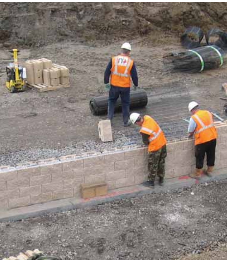
Keystone® blocks are delivered on pallets to the point of installation.
