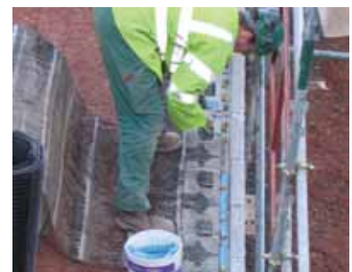
A feature common to the Tensar tech Keystone® Wall System is the high efficiency connection between geogrid and facing unit, which is quick and easy to secure.
