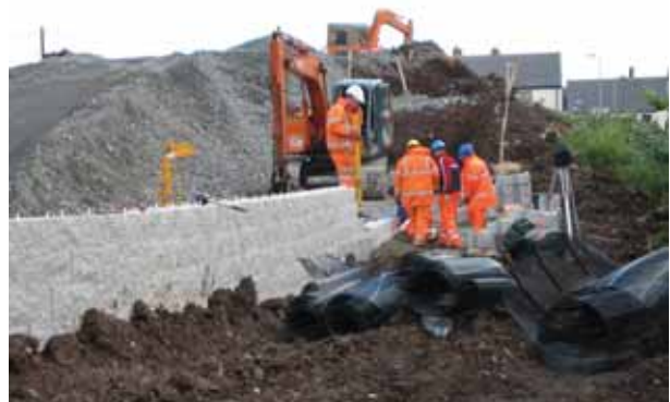
This project demonstrates that the Tensar tech Keystone ® Wall System can be built without cranes or propping.
