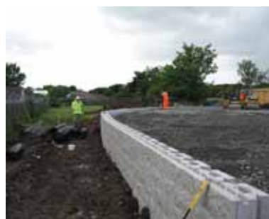
Keystone® Facing units are simple to install and can easily accommodate tight concave or convex horizontal curves.
