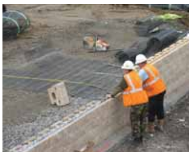
The Keystone® concrete blocks and Tensar geogrids are simple to install.
